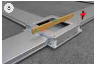
8 Make the level adjustment on scales of the junction box.
