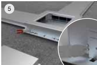
5 Cut the separator plate based on duct dimension.
