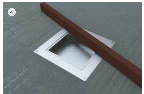
11 Apply the levelling screed. Fill completely without any empty sections under the duct and junction boxes.
