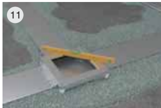
11 Apply the levelling screed. Fill completely without any empty sections under the duct and junction boxes.
